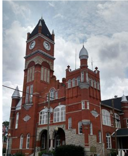
Terrell County Courthouse, circa 1892
