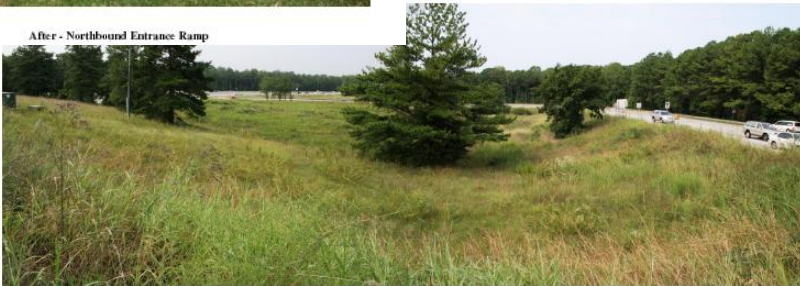
Before - Southbound Exit Ramp Loop
